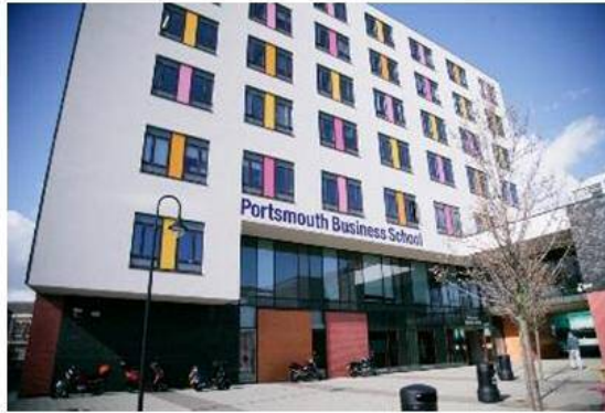
Richmond Building (RB) , Portland Street, PO1 3DE
