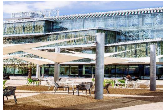
Portland Building (PO) , Portland Street, PO1 3AH
